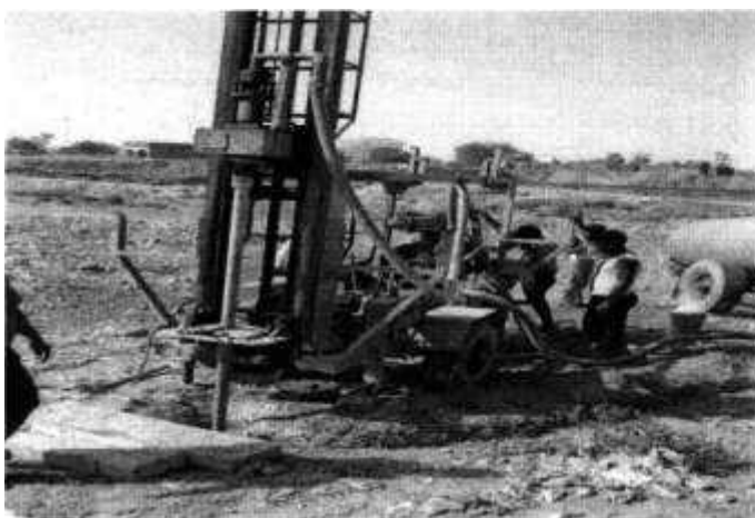
Step iii): Mode of drilling using Direct Circulation System Rotary (Mud Rotary Drilling) method
